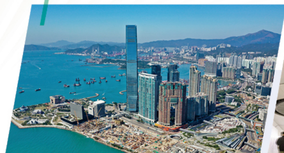
Infrastructure at West Kowloon Cultural District
