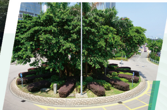
Roundabout at Man Kwong Street / Man Yiu Street
