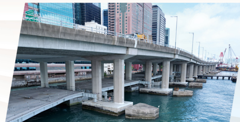
Boardwalk under Island Eastern Corridor
