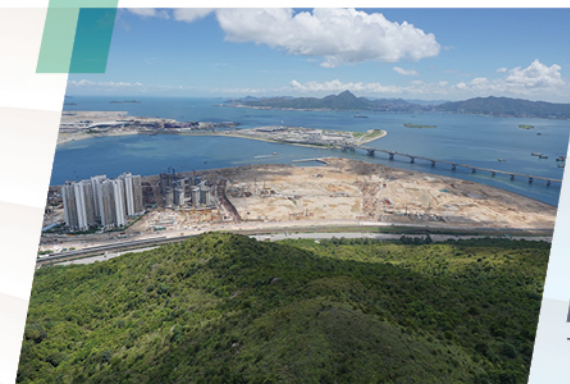
Completion of Reclamation Works in 2023
