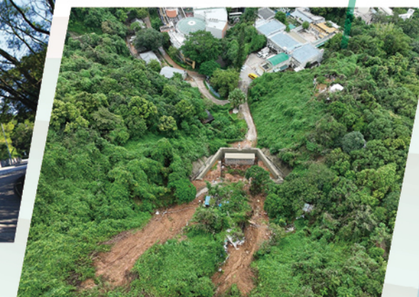
Rigid Barrier at Pinehill
