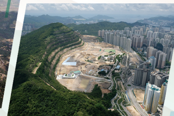
Anderson Road ( After Construction )
