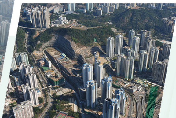
Choi Wan Road and Jordan Valley ( After Construction )
