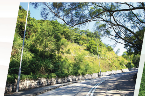
Stabilised Natural Slope
