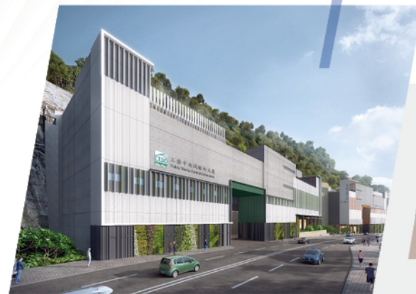
Joint Cavern Development
