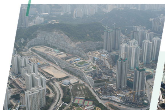
Choi Wan Road and Jordan Valley ( Before Construction )
