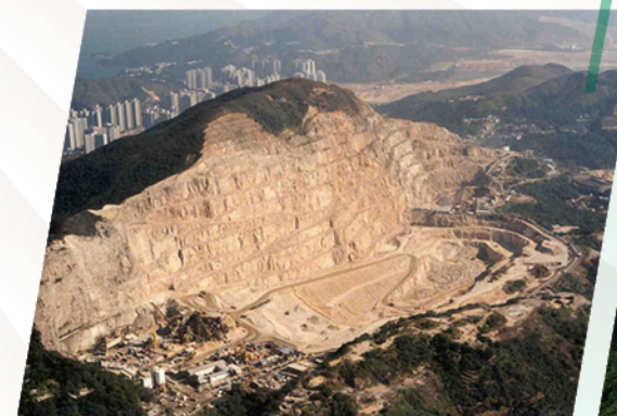
Anderson Road ( Before Construction )
